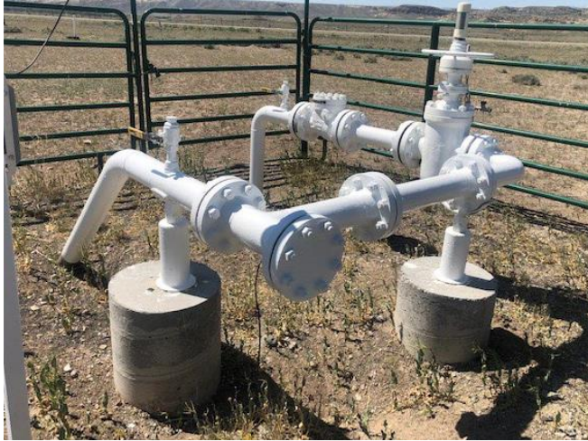
Figure 5--Launcher Site with No Trap Installed
