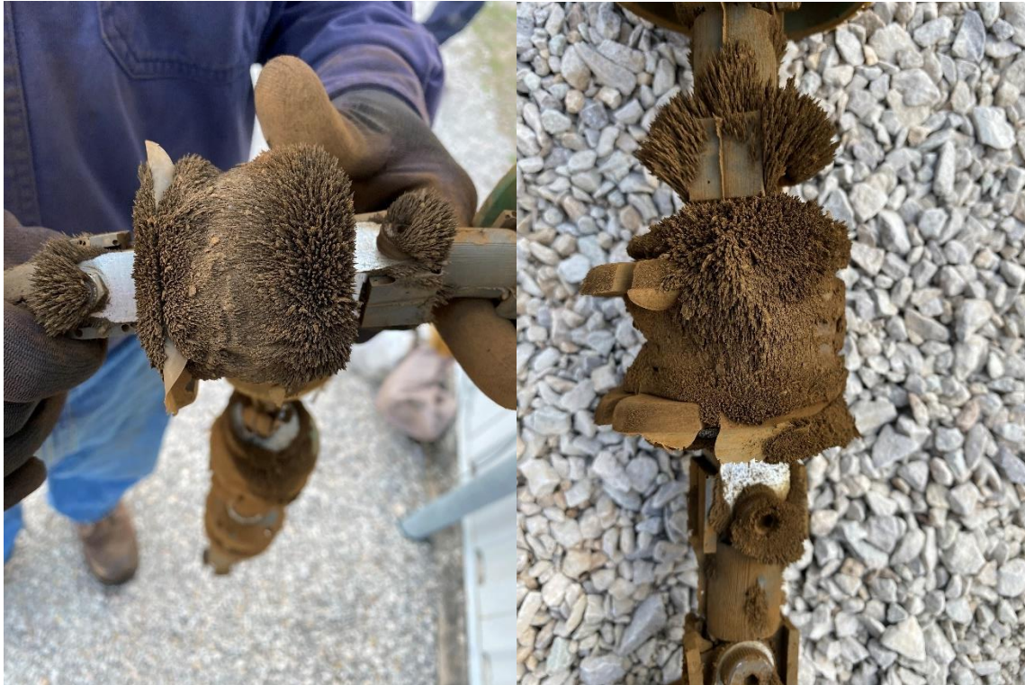
Figure 19--Magnetic Cleaning Pig Results, with Ferrous Debris Attached to the Magnet
