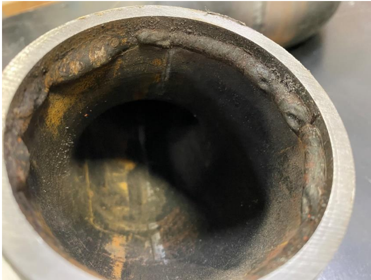
Figure 3--Heavy Weld Penetration at Transition from Straight Pipe to 1.5d Bend
