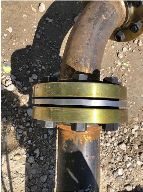
Figure 3 Flange with Restriction Ring
